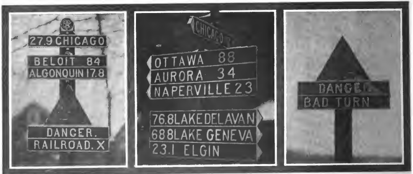
Some of New Signs—At Railroad Crossing, Elaborately Marked Intersection, Dangerous Turn
